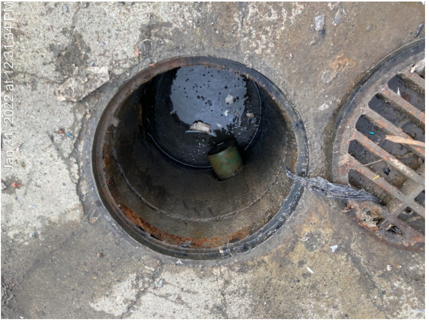
Photo 3. View of the Storm Drain within the GFL Facility.
