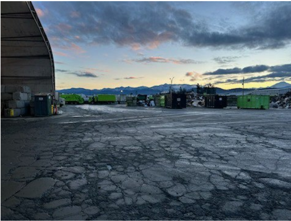
Photo 3. View of the significant asphalt cracking.
